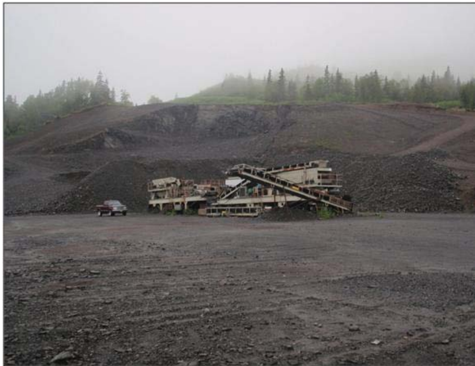
Figure C - 28. View of Ekuk Quarry Production Face, Crusher, and Screens
