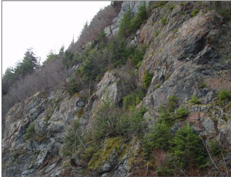
Figure C - 31. Existing Rock Ledge Adjacent to the Sitka Highway
