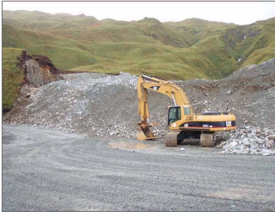
Figure C - 3. View of Bering Shai Quarry from Staging Area
